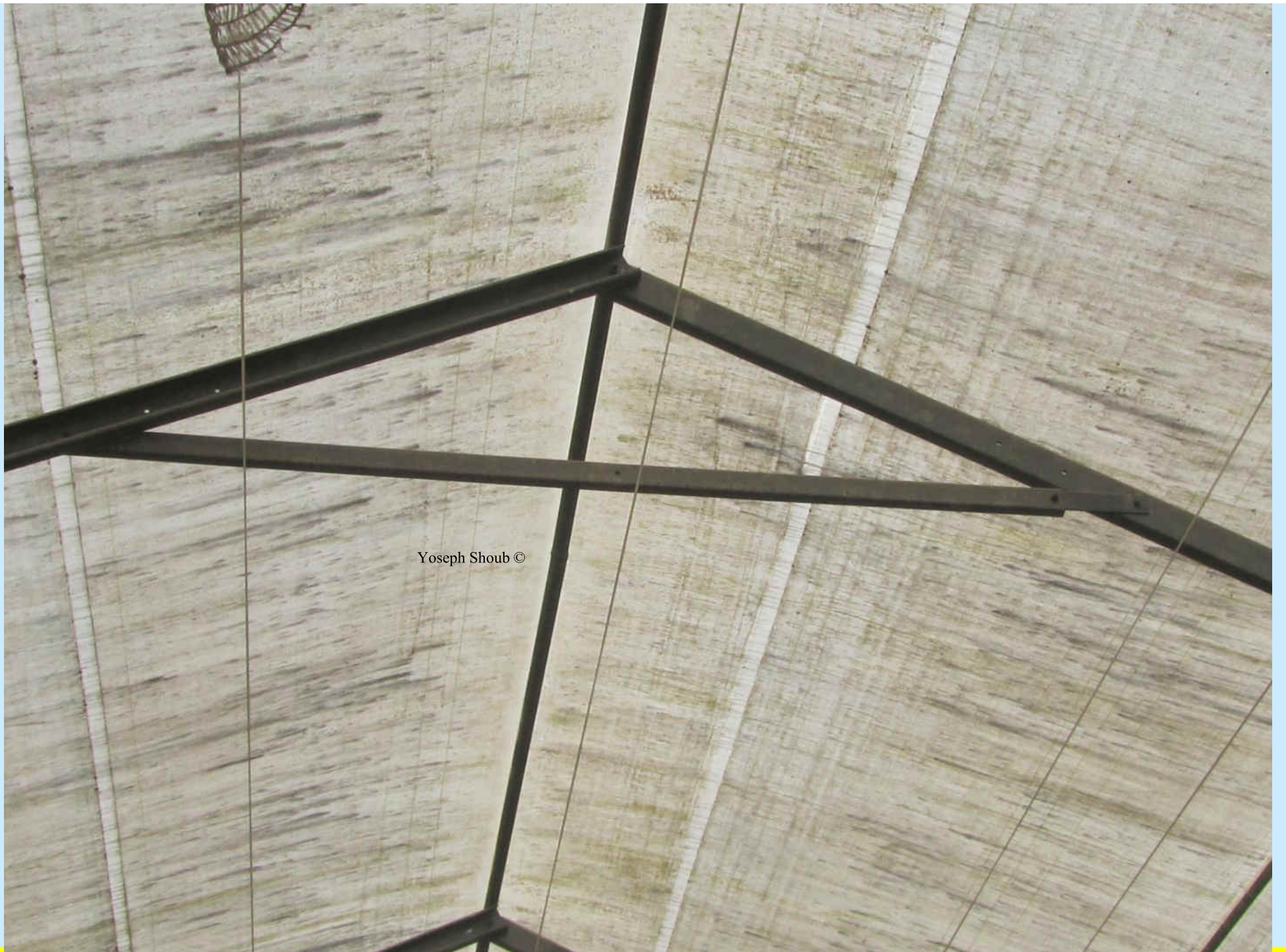
8 Years old P.E. (“Palrig“ cloth), reduced the light radiation in our greenhouse through 2017 / 2018 season.
